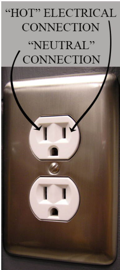
“Wall” outlet provides 120 V RMS ac voltage between the “Hot” and “Neutral” connections.
